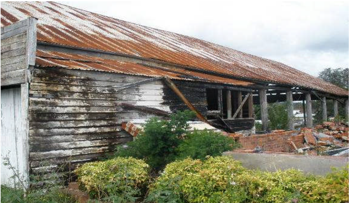
Photo 18. Fire affected weatherboards
