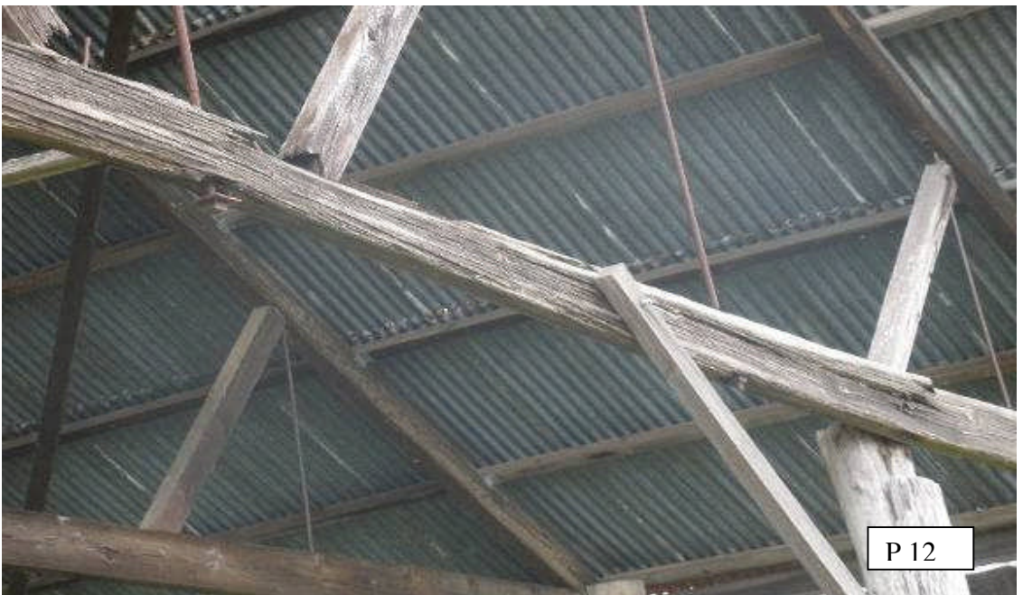
Photo 14. Eastern End Failed Truss (P11-P14) immediate remedial works required
