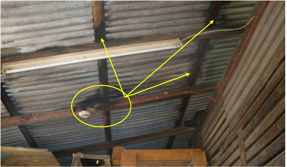
Photo 18. Fire affected weatherboards
